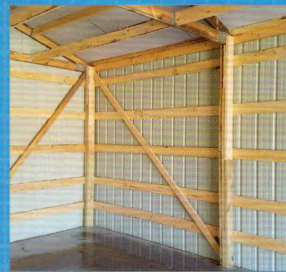
2' On Center Girted Walls
